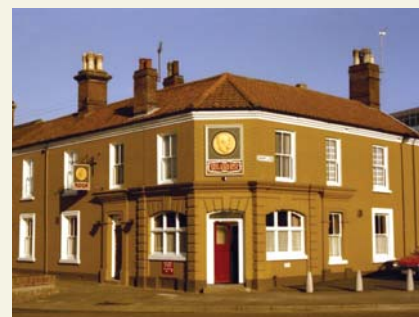
The Victorian former Cherry Tree pub at 43–45 Pitt Street in 1970, which is locally listed (Credit: Martin Hooker)
