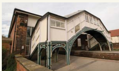
Footbridge at Beverley Railway Station (Credit: Alamy)
