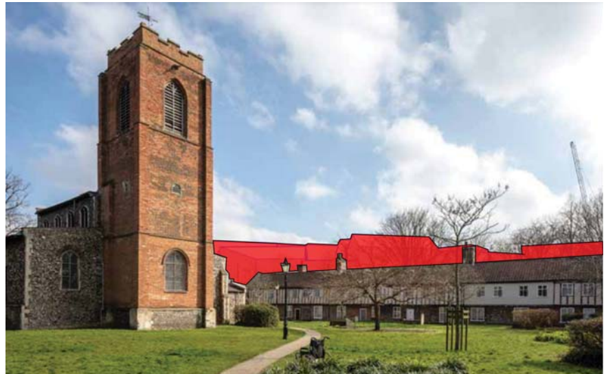
View of the new proposals (in red) which would be highly visible from St Augustine’s churchyard, a historically sensitive part of the city centre conservation area (Credit: Montage by SAVE based on planning documents)
