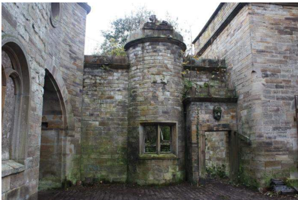
Below: The same view cleared of plant growth, in 2014
