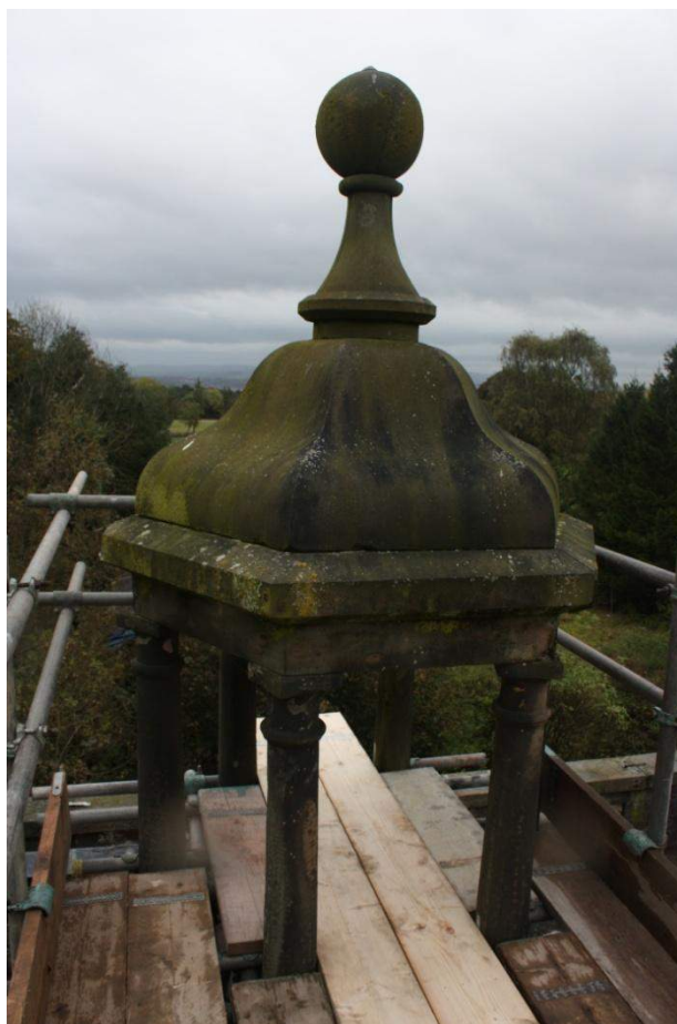
Above: One of the cupolas being restored in situ
