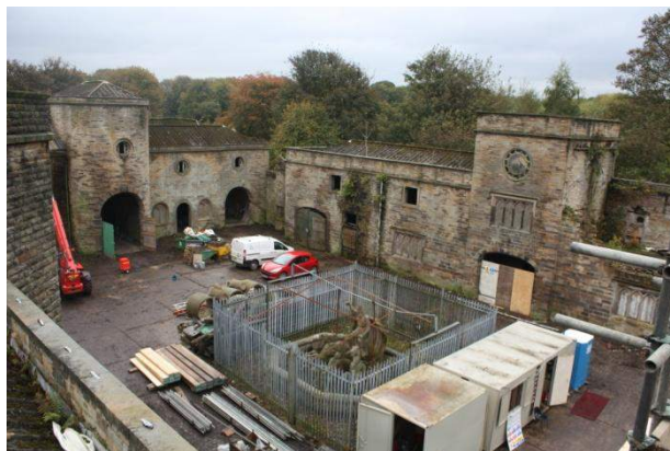
Above: The stable courtyard being cleared of plant growth
