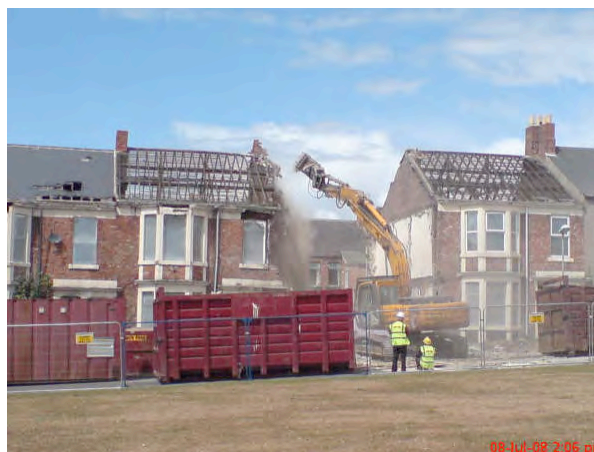
Demolition contractors get to work in Gateshead
