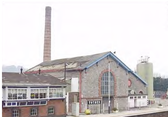
Brunel's pumping station at Totnes, Devon
