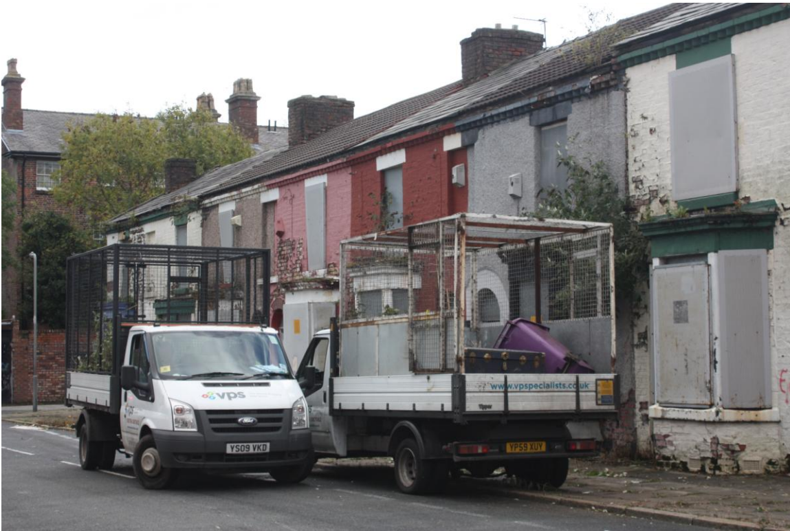
Management companies at work on the Welsh Streets, who are paid to keep the streets clear and the deteriorating properties bolted, but not to repair them.
