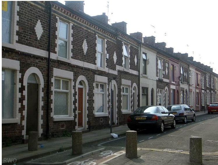
Above: Vienna Street, Anfield, 2007. Demolished 2014.
