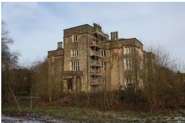
Repairs to one of the chimney stacks on the main house
