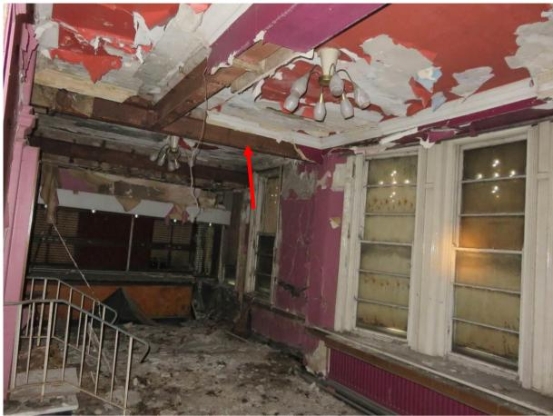
Photograph 3: First floor room with steel beams spanning front elevation back to the cross wall behind
