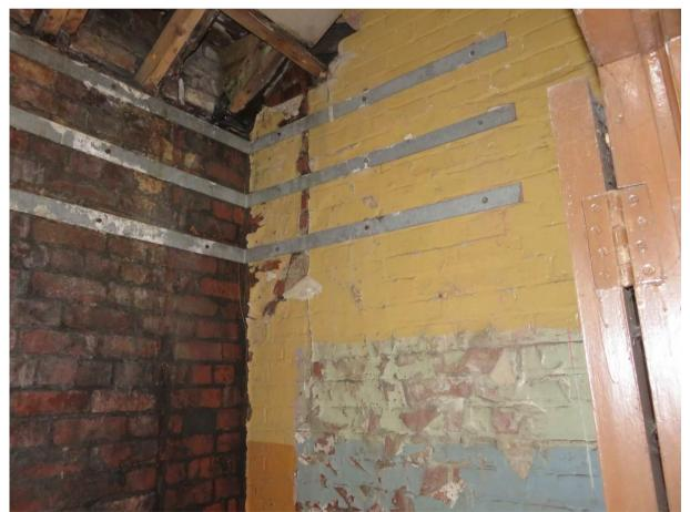
Photograph 2: Cross wall with temporary restraint straps
