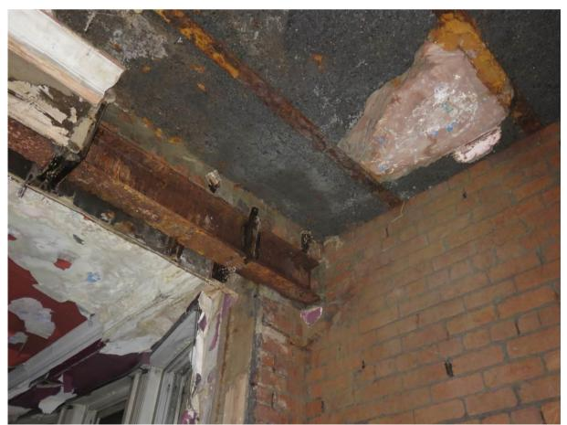
Photograph 4: Steel beam to front elevation with no evidence of corrosion jacking to built-in end
