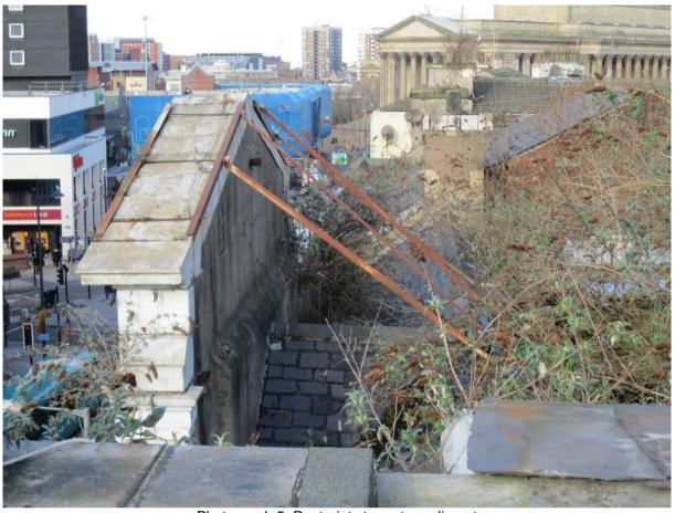
Photograph 5: Restraint straps to pediment
