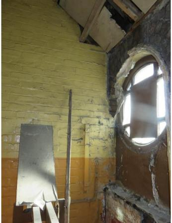
Photograph 1: Cross wall to front elevation providing lateral restraint and with no evidence of cracking
